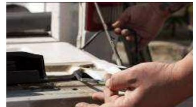
If you feed the bottom portion of our harness up through the tailgate you can use it to pull the of the wires down through the tailgate.
