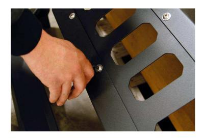
**2.** Install the Fab Fours Vi-Cowl windshield brackets using OEM hardware. Finger tighten all bolts first then fully tighten.
